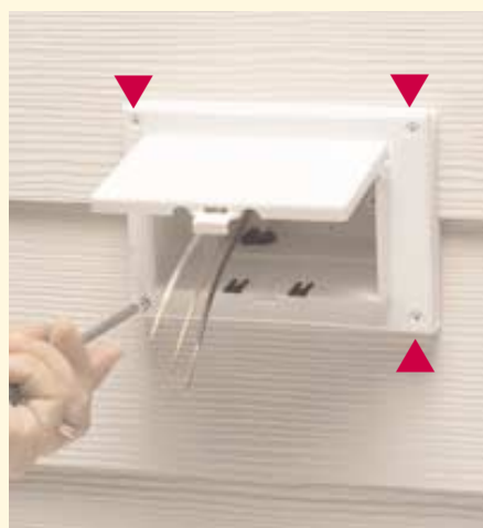
3. Apply caulk to reverse side of IN BOX flange. Install NM cable connector and wire, then attach with long screws (provided). Trim excess caulk as needed. Install wiring device.
