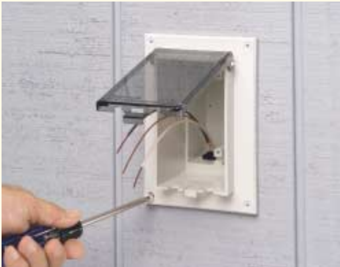
3. Attach IN BOX with stainless steel screws (provided).
