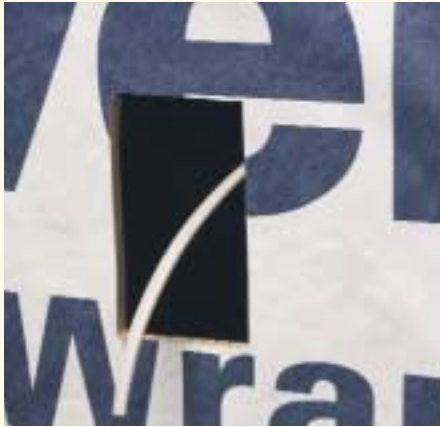
1. Cut hole in substrate. Pull wiring.
