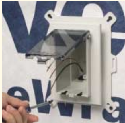
2. Install NM cable connector and wire... attach IN BOX to substrate.
