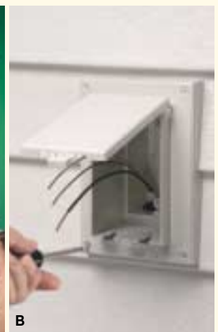
3A. Apply caulk to reverse side of IN BOX flange.
