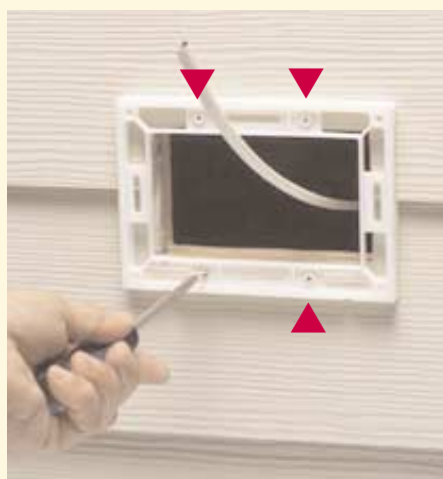
2. Apply caulk around edges of back of adapter (see page 7 for photo guide). Press onto siding. Attach adapter to siding with (supplied) short screws through the holes noted above. Trim excess caulk as needed.
