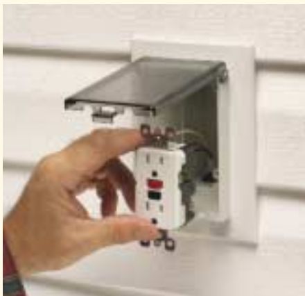
4. Install wiring device.
