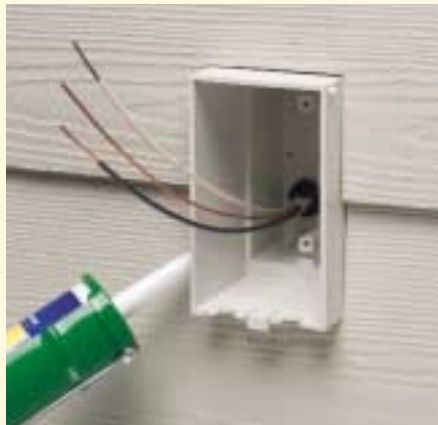
3. Cut rigid siding to fit around IN BOX . Caulk around box.
