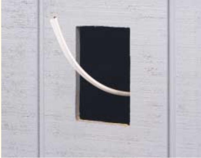
1. Cut hole. Pull wiring.
