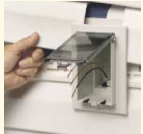
3. Install siding, inserting the cut ends of the siding under the outer flange of the IN BOX .
