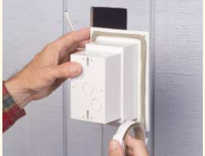
2. Apply the supplied caulk around back edges of flange. Install NM cable connector and wire, then press onto surface.
