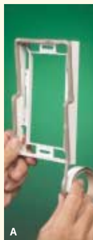
2A. Apply caulk around edges of back of adapter. Press onto siding.
