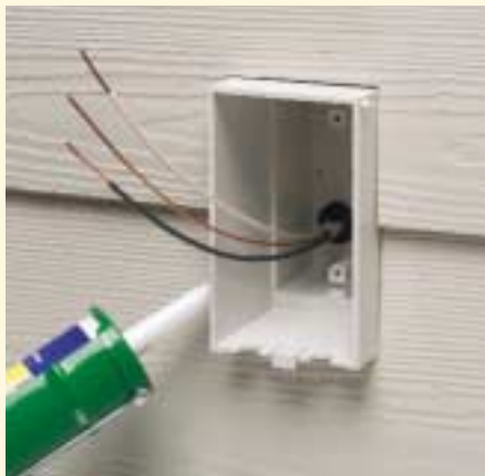
3. Cut rigid siding to fit around IN BOX . Caulk as above for a great looking job!
