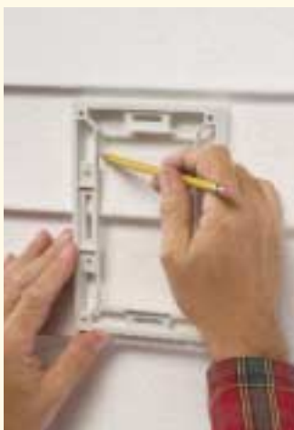
1. Using the siding profile adapter plate as a template, cut hole in existing siding. Pull wiring.
