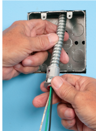
Snap fitting onto cable.
