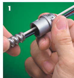
Snap fitting onto cable... twist clockwise
