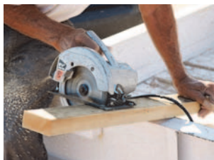
Construction Site Application
