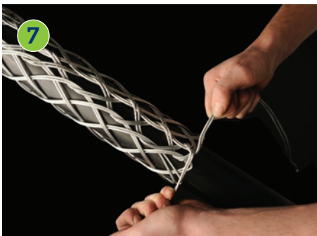
Finally, tie the ends of the lace once or twice round the end of the cable grip twisting the ends together securely. Excess lace can be cut off.
