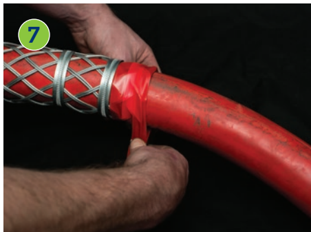
Tape should then be wound around the end of the cable grip furthest away from the eye ends.
