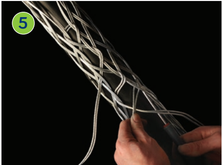
As you continue down the length, pull the open sides of the grip as wide apart as required.
