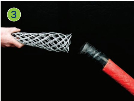
The grip should then be placed over the end of the conductor...
