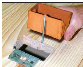
Install clip over subfloor.
